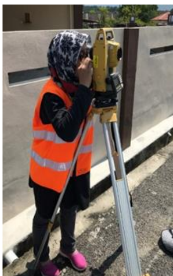
Figure 6. Total station survey
