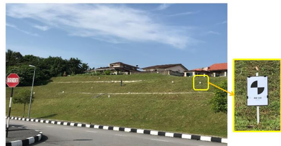
Figure 2. The landslide area with the well-distributed measurement targets
