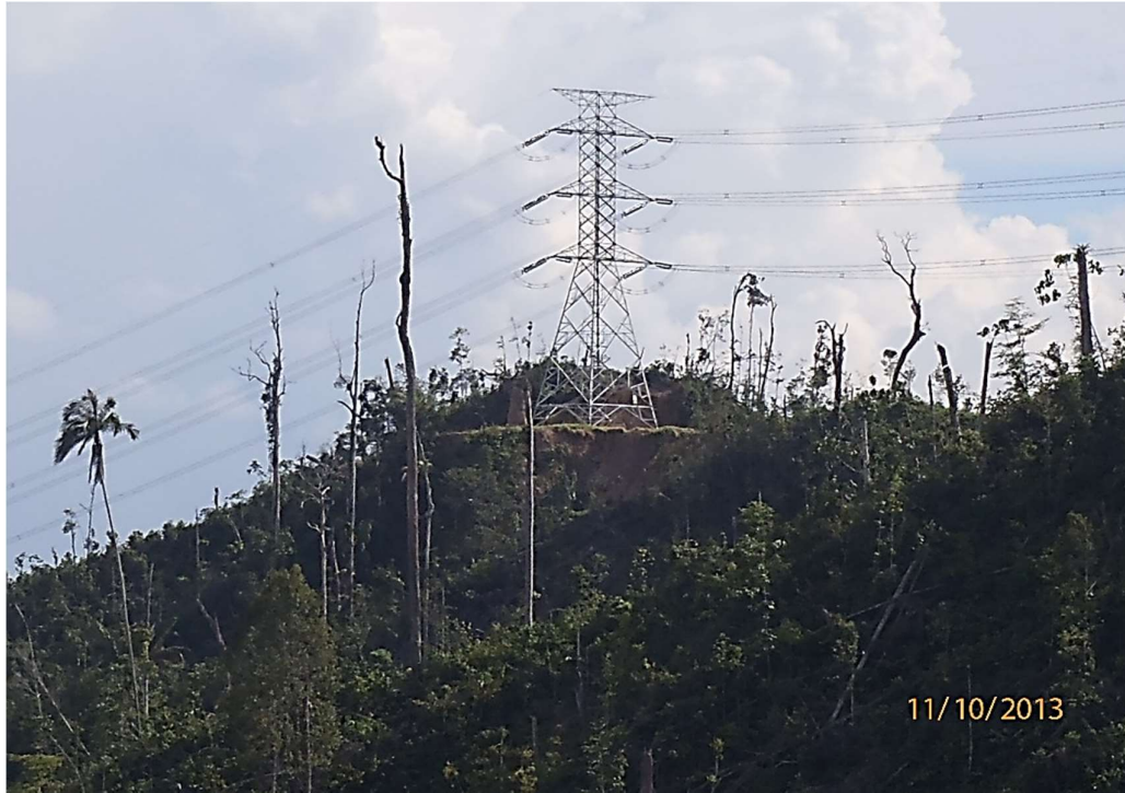
Figure 1.2 Transmission tower constructed on top of slope
