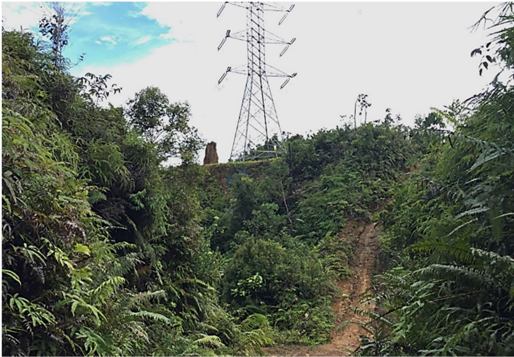
Figure 1.3 View of MJM 117 from bottom
