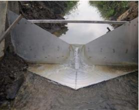
Figure 3: 120° V-notch weir
