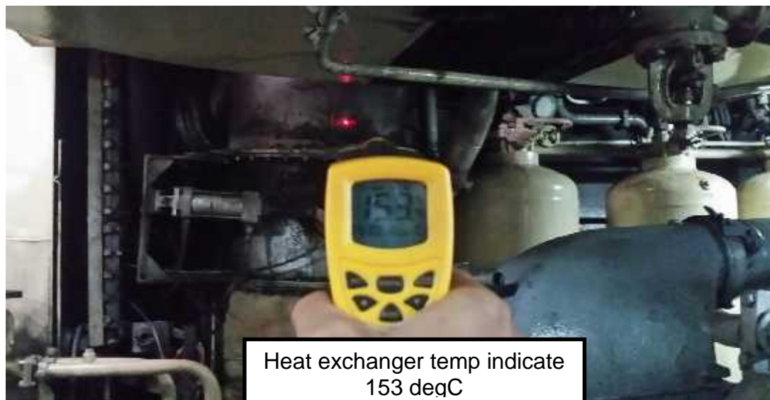
Figure 1.4: Exhaust Heat Exchanger Temperature
