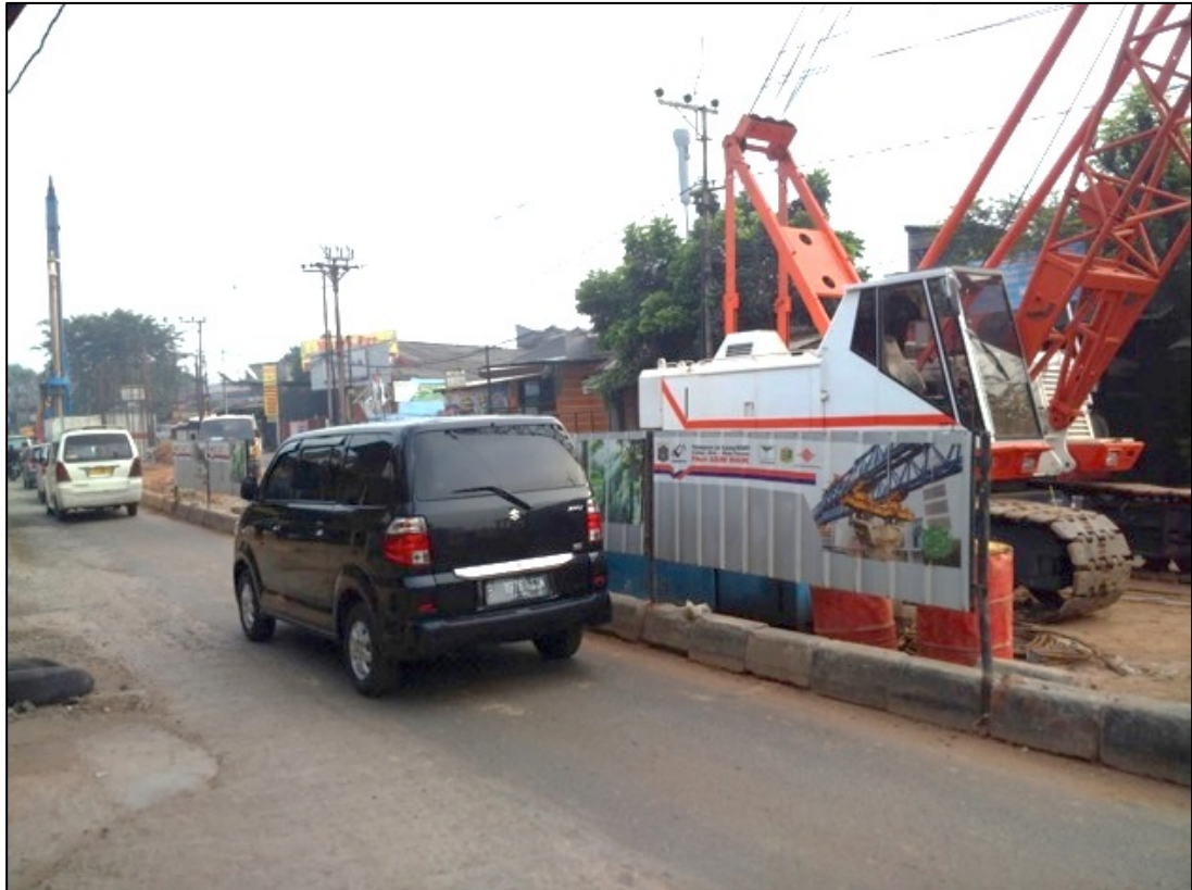
Figure 1.4 Construction of flyover project adjacent to dense traffic, Jakarta
