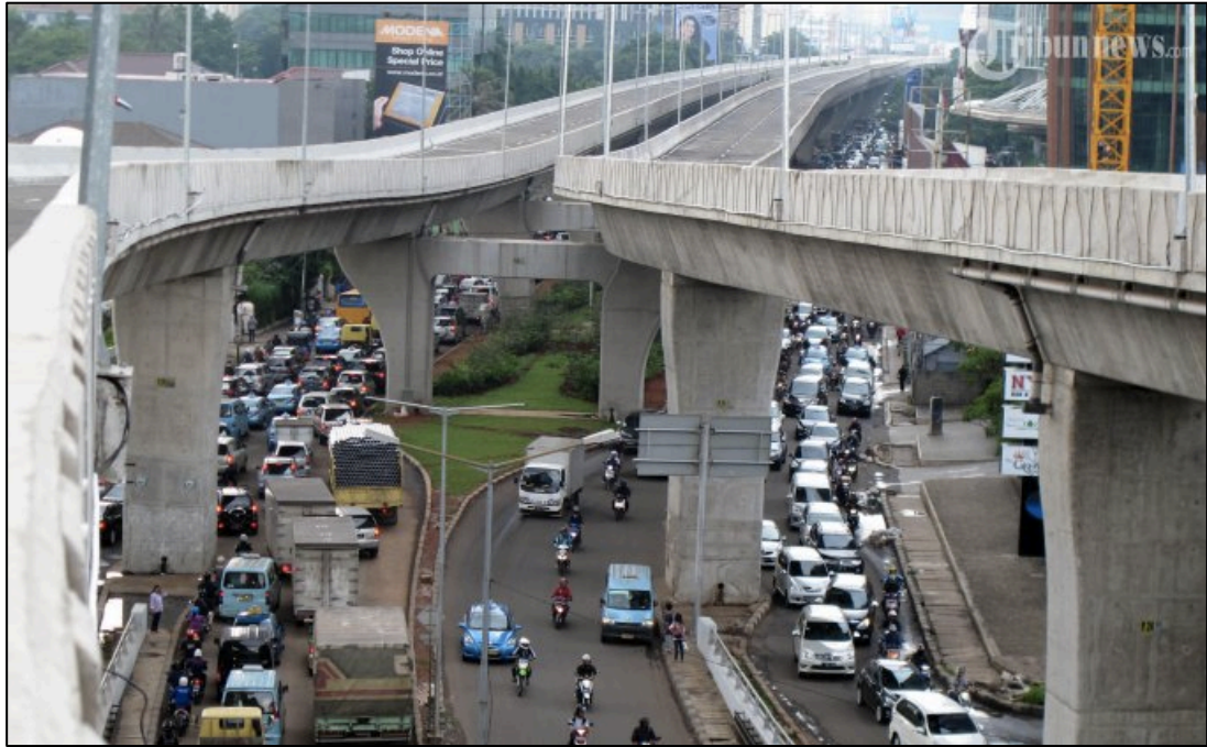
Figure 1.3 Kampung Melayu – Tanah Abang flyover with existing road below, Jakarta
