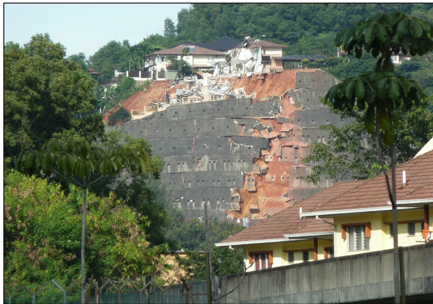
Figure 1.1 Front view of the slope failure
