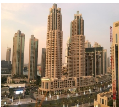
Figure 1: Vertical constructions for maximum utilization of land 29 Bulivard: construction completion date 1976 (Source: Authors)
