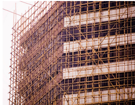
(b) Bamboo Scaffolding [6]
