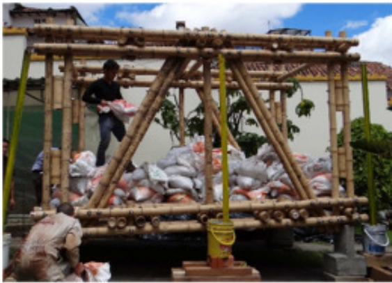
(a) Footbridge Prototype [5]
