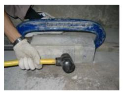
Figure 3: Hacking with air tool hammer
