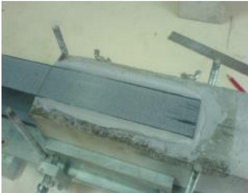
Figure 7: Bonding CFRP Plate to concrete
