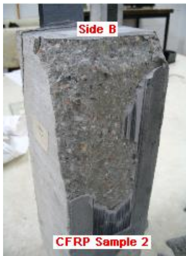
Figure 16: Typical brittle bond failure for CFRP/Con 2
