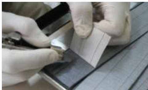
Figure 5: Peeling CFRP plate protective layer
