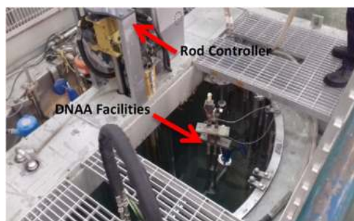
Fig. 1. The top view of TRIGA PUSPATI reactor pool.
