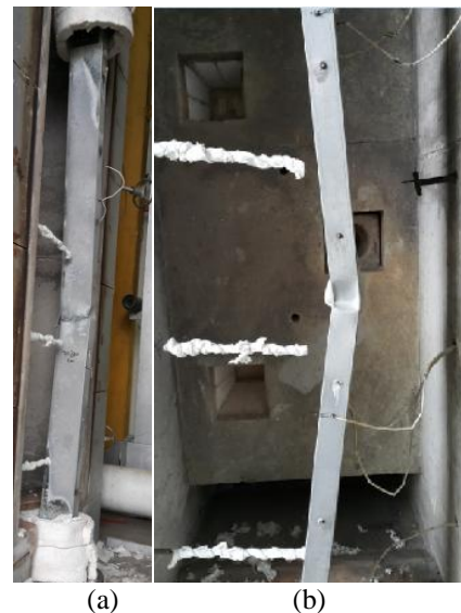
Fig. 9 (a) Test set-up (b) buckling of box-up column
