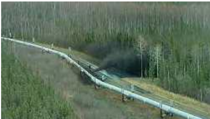
Figure 1.2 Gas leakage on natural gas pipeline (courtesy of Doug, 2014)
