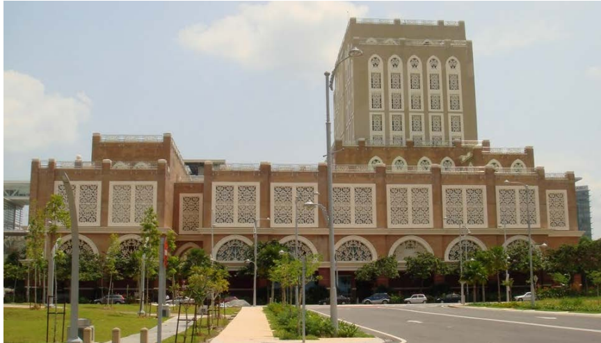
Figure 1.1 Building of Legal Affairs Section (BHEUU)
