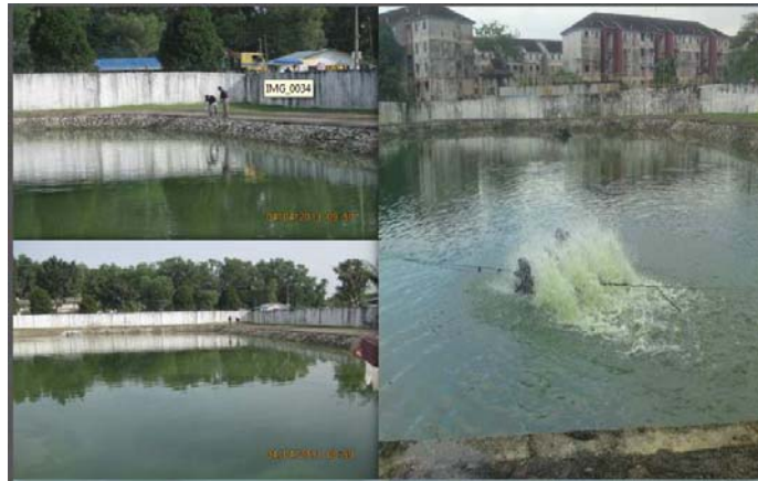
Figure 1.3 Physical Condition of Oxidation Pond, Tampoi, Johor Bahru [3]
