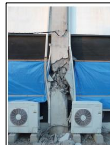
(b) Structural (column)
