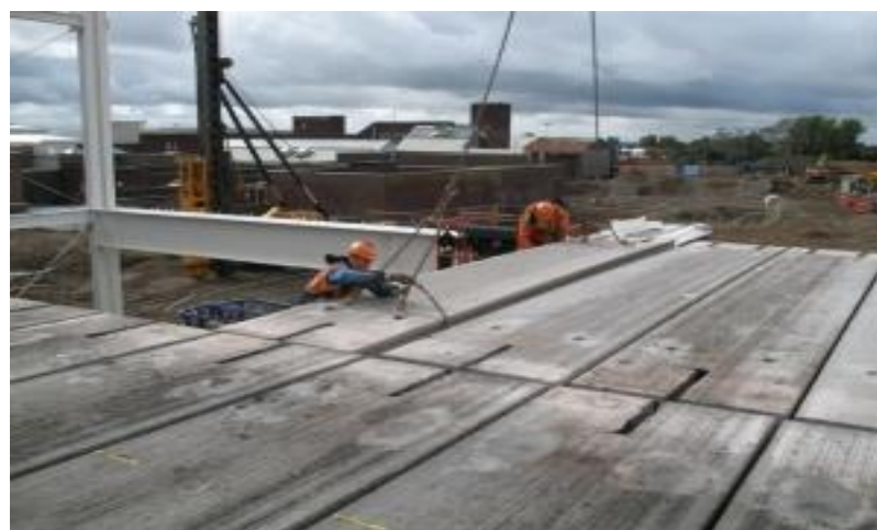
Figure 1.1 Placing the precast slab
