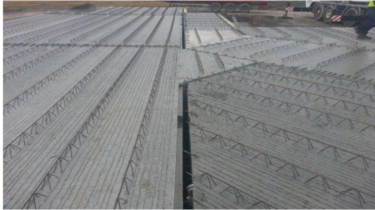
Figure 1.3 Projecting steel at the top of the precast slab
