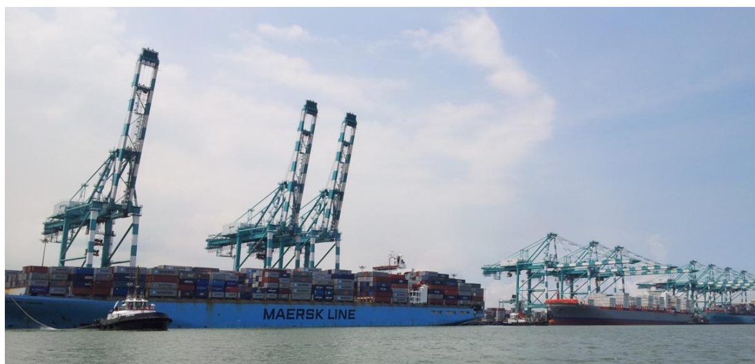
Figure 1.2 Shipping transits at Pulai River Estuary
