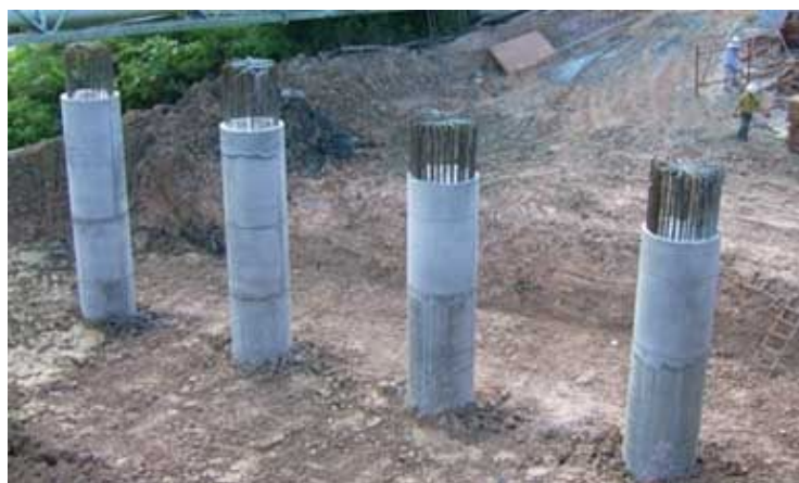
Figure 1.1 : Bored Pile
