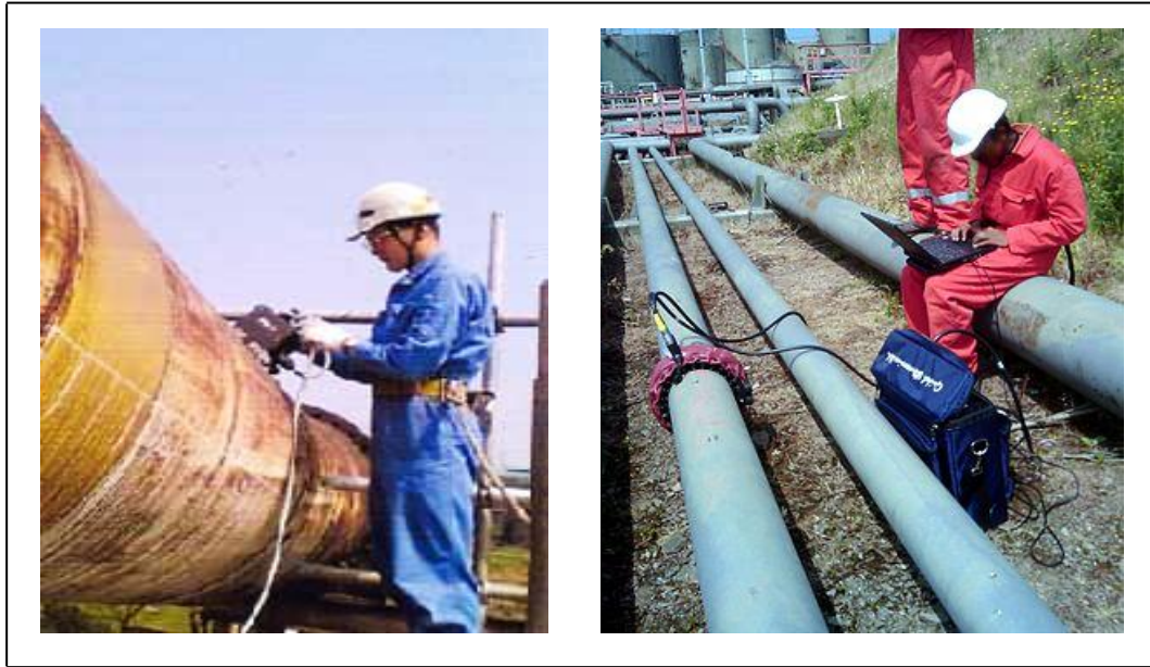
Figure 1.4 Varies of pipe inspections (Zhang et al. , 2007)
