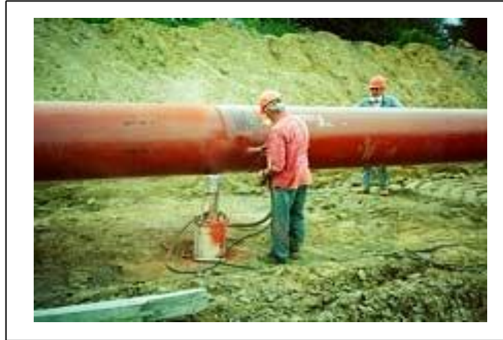
Figure 1.2 Pipeline coating (Beller et al. , 2001)
