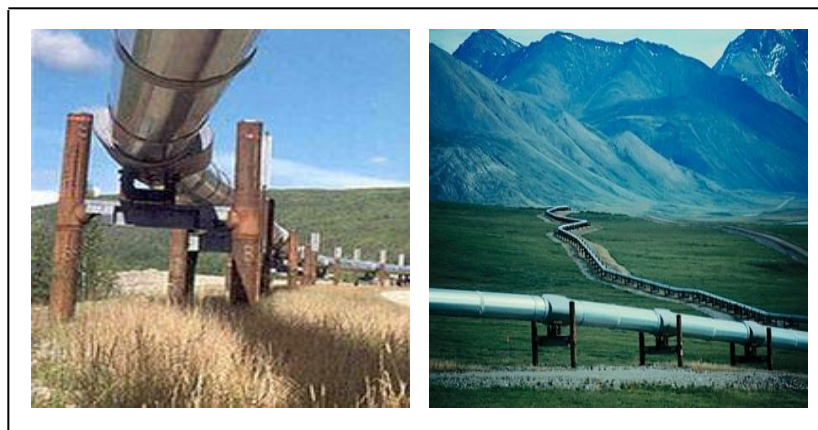
Figure 1.1 Oil and gas pipeline (Bonny et al. , 2008)
