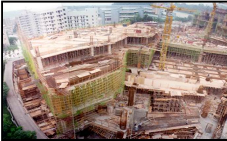
Figure 1.2 The view of site construction that uses traditional timber formwork.
