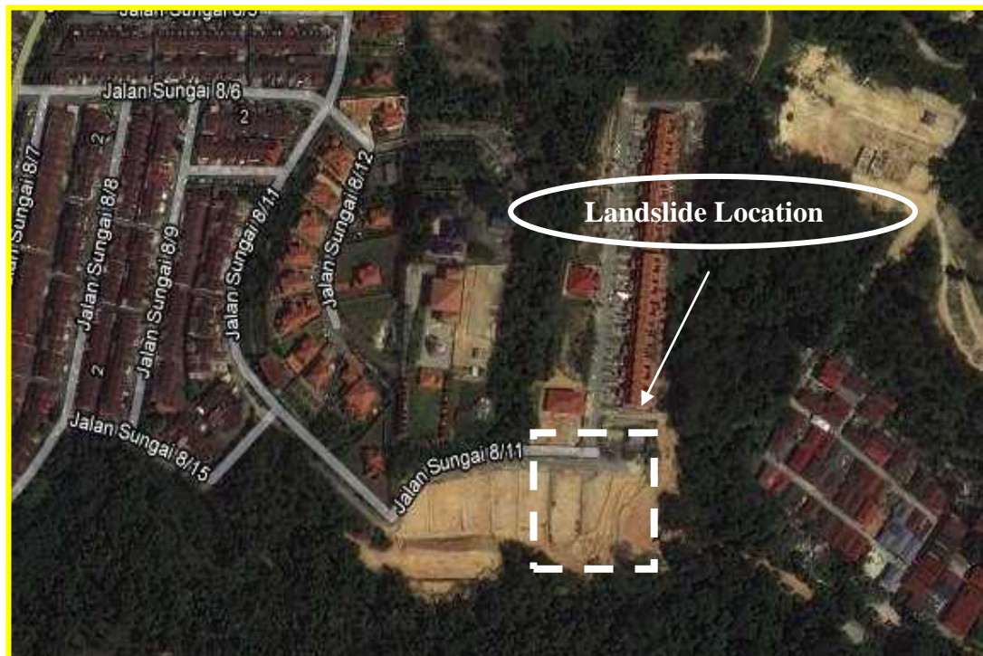
Figure 1.1: Aerial view of site location showing landslide area
