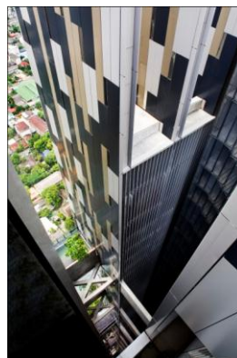
Figure 1.8 The Met – Bangkok by WOHA (2013), view looking down through the semi-enclosed lightwell between the towers, (Source: Feng (2012))
