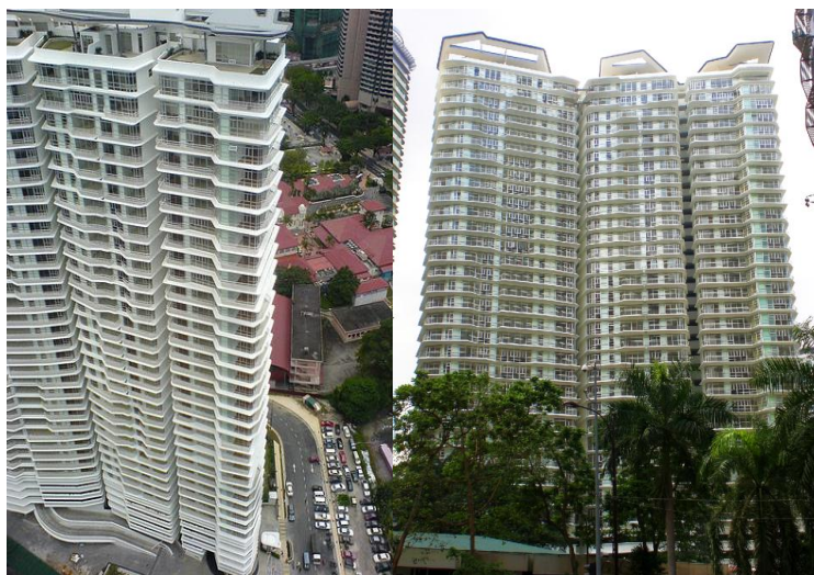
Figure 1.5 The Idaman Residence - Kuala Lumpur by T. R. Hamzah & Yeang (2008), using semi-enclosed lightwells as funnels to capture wind, wind corridor and attached lightwells (Source: http://www.skyscrapercity.com )
