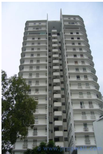
Figure 1.4 The Residence - Kuala Lumpur by T. R. Hamzah & Yeang (2006), attached lightwell, wind corridor and wing-wind wall (Source: http://www.propwall.my )
