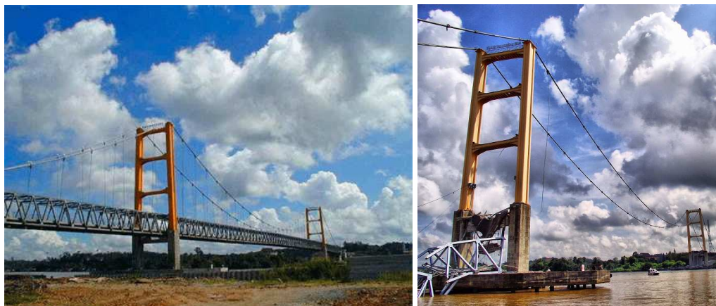
Figure 1.2 Kutai Kartanegara Bridge before and after collapse (JPCL, 2012)
