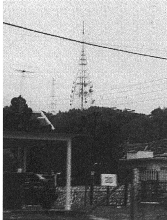
Fig. 1. Observed telecommunication station.
