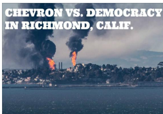
Figure 1.8 Explosion and fire caused by leakage in a 1.5m 8-inch carbon steel pipe suffering from sulphide corrosion – HTM PSM Case Reference
