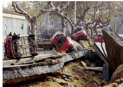
(b) Qingdao city oil pipeline leak (The Telegraph, 2013)
