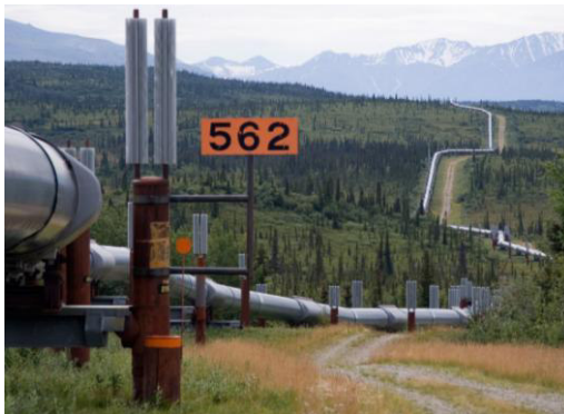
(a) Trans-Alaskan oil pipeline leak (The Guardian, 2011)
