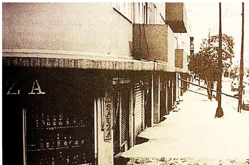
Figure 1.3 Settlement of a building in Mexico City due to ground subsidence phenomenon during the 1985 Michoacán earthquake (Villaverde, 2009)
