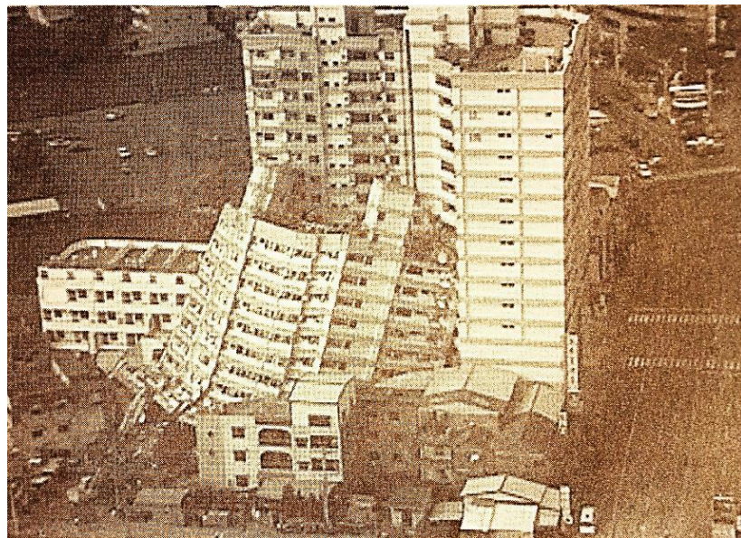
Figure 1.2 Collapse of middle rise building during the Chi-Chi earthquake in 1999, Taiwan (Villaverde, 2009)
