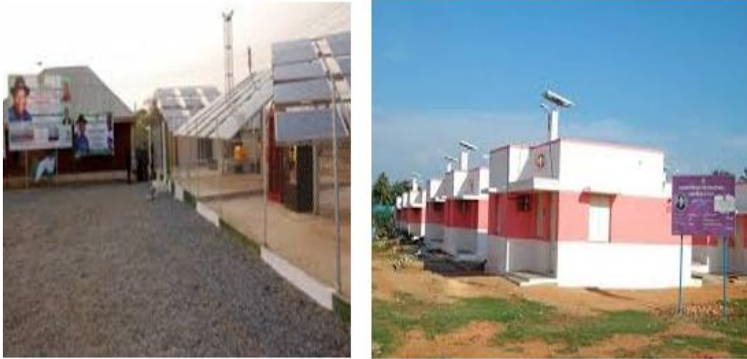
Figure 1.1 Installed solar power system at Idda village, Kogi state [12].
