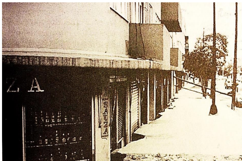
Figure 1.3 Settlement of a building in Mexico City due to ground subsidence phenomenon during the 1985 Michoacán earthquake (Villaverde, 2009)
