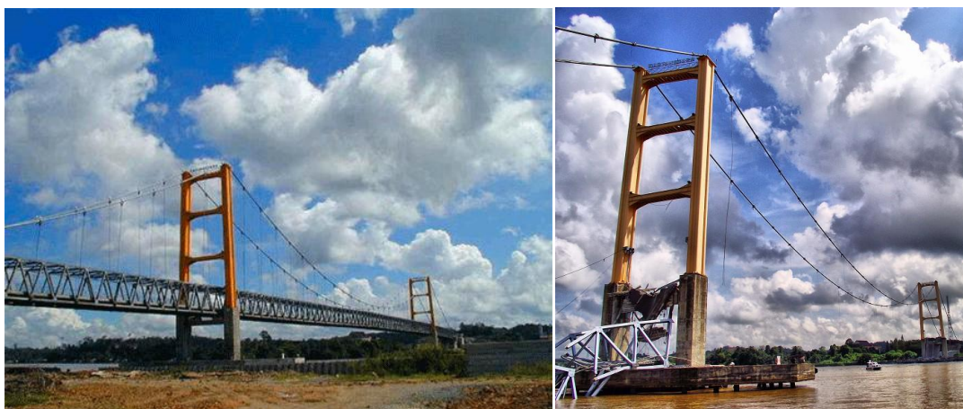
Figure 2. Kutai Kartanegara Bridge before and after collapse [7]
