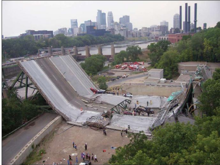
Figure 1. One section of the I-35W Bridge collapse [6]
