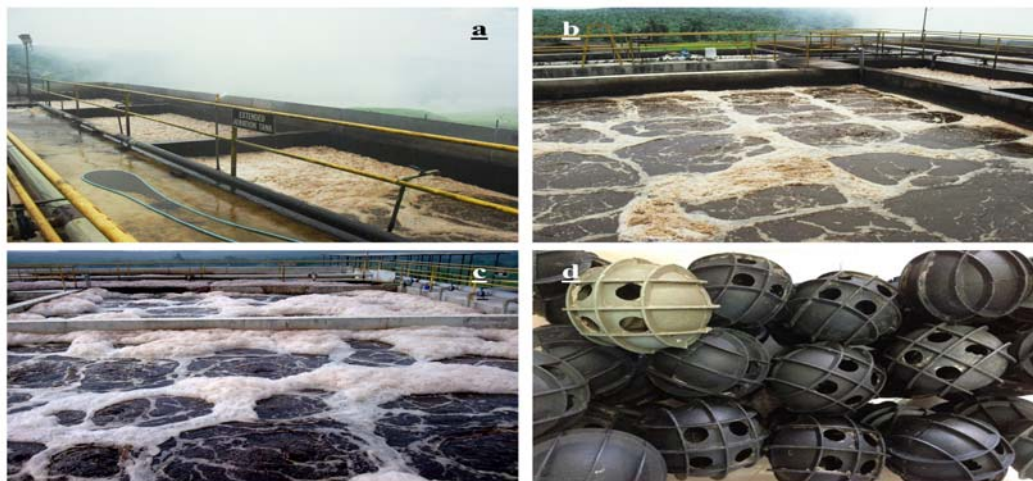
Figure-1. The IETS (IETS-3) showing overall highest removal efficiencies of BOD and nutrients. The polishing system consists of (a) extended aeration, (b) & (c) fixed packing media submerged in the activated sludge aeration tank, and clarifiers before final discharge. (d) showed the plastic media used in the IETS.
