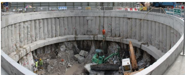
Figure 9 Circular shaft during excavation.
