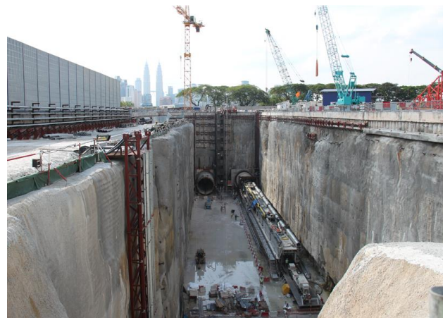
Figure 16 Cochrane Station (launching of second TBM).
