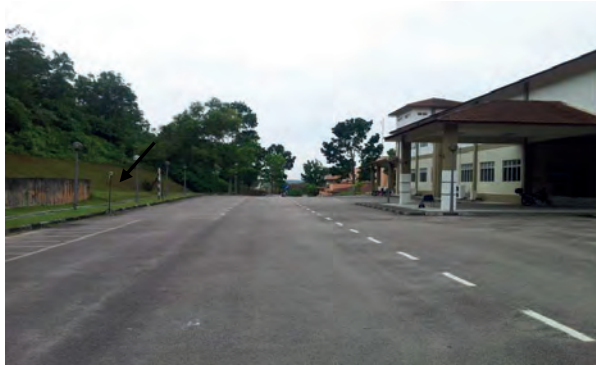
Figure 3. Environment A: roadway measurement environment.
