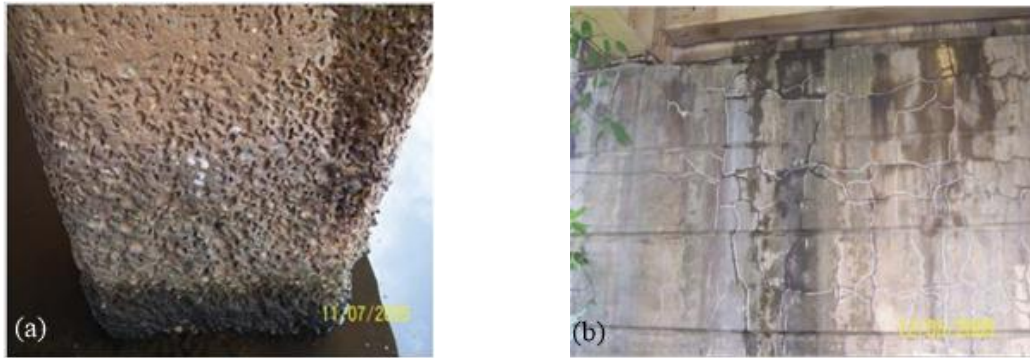
Figure 1 Problems to bridge components (a) Acid attack on limestone aggregates (b) Map Crack due to AAR at the abutment of Tamparuli Bridge [7]
