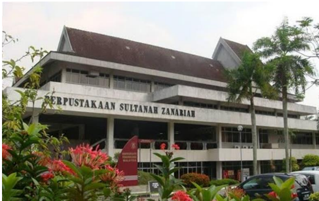
Figure 2 View of the library building
