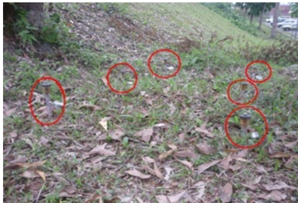
Figure-1. Tensiometer installed at toe of slope.
