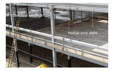
Figure 1 Concrete toppings on hollow core slabs
