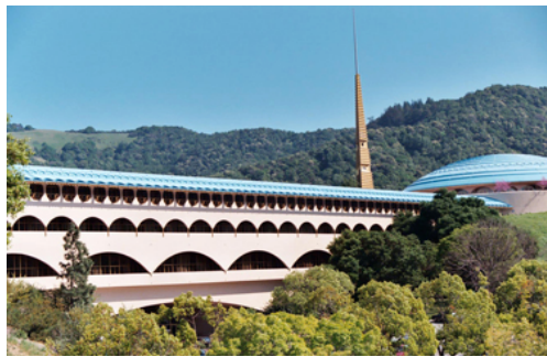
Figure 1: Marine County Civic Centre Tower (Meehan 1987; 366)
