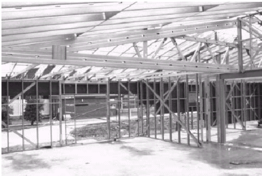
Fig 2 Cold formed steel framing (light steel framing) for residential house in UK (Adopted from Grubb, 2001)
