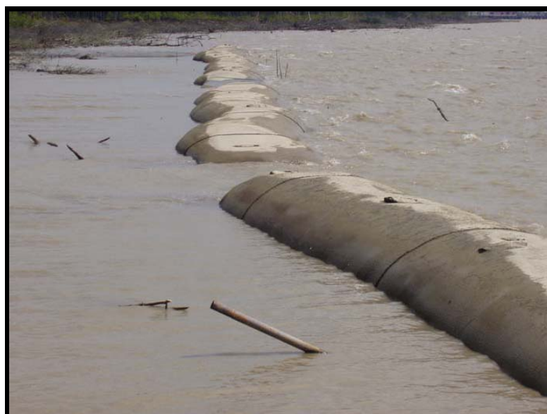
Figure 1.1: Geotubes installed at Tanjung Piai (Source: JPS, 2005)
