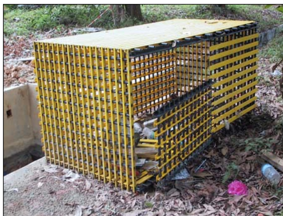
Figure 1.1: The mesh type rubbish and sediment trap
