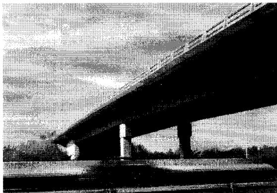
Figure 1.7 : Asterix Bridge , A1 Motorway Interchange, France
