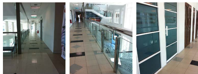
Fig 4: The corridor at Section B., plasterboard wall, the clear glass barrier, tinted glass door and wooden door.
