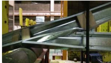
(b) Failure of the roof truss at maximum load applied at front view
