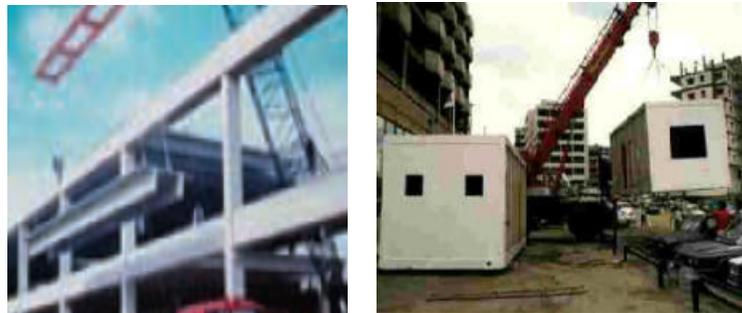
Figure 2.1: Precast Concrete Framing, Panel and Box Systems
