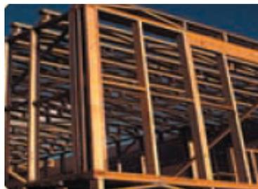
Figure 2.4: Prefabricated Timber Framing Systems
