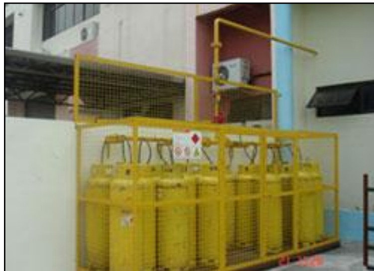
Figure 1.2 Manifold LPG system (Primagas, 2009)
