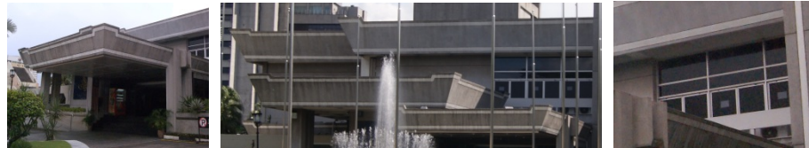
Layer 6 (Simple use of detailing and elements on façade)
