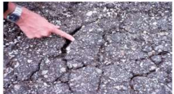
Figure 4 Fatigue cracking [3]
