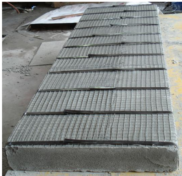
Figure 5.21: Wall elements with steel strips
