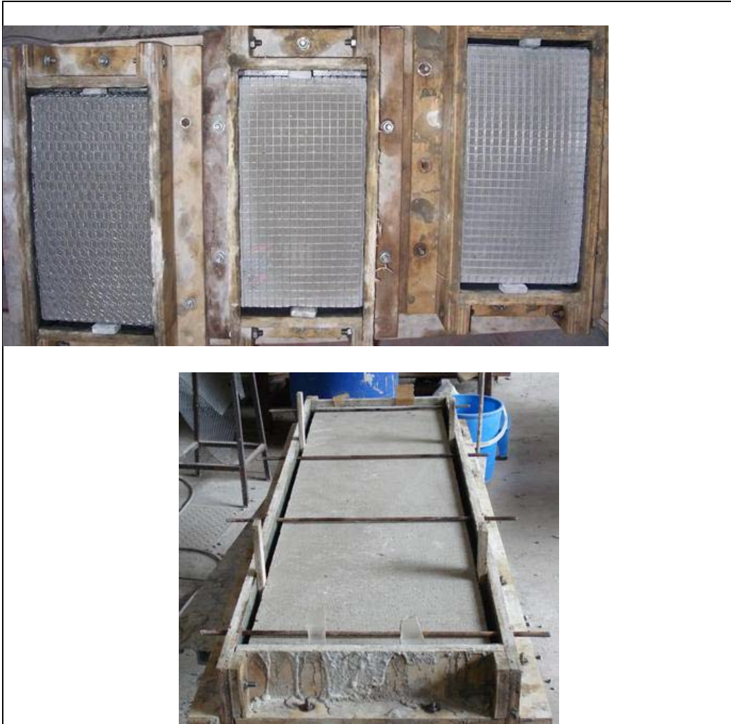
Figure 3.20: Sandwich specimens ready to cast encasement
