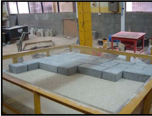
Figure 3.14 Installation of CBP
