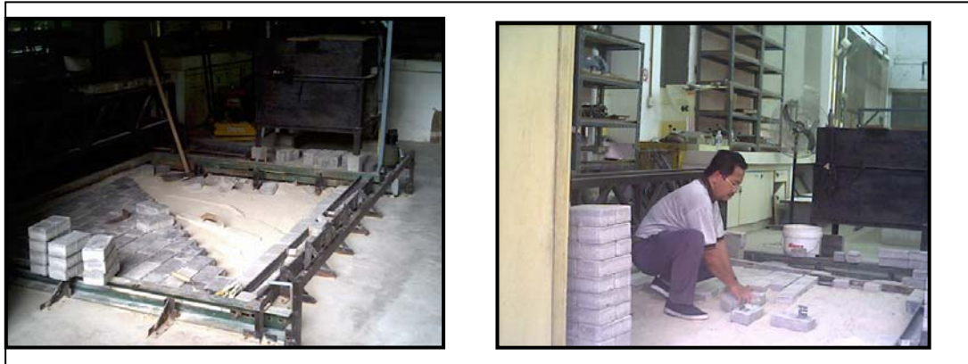
Figure 3.8 Installation of concrete block pavement (CBP)
